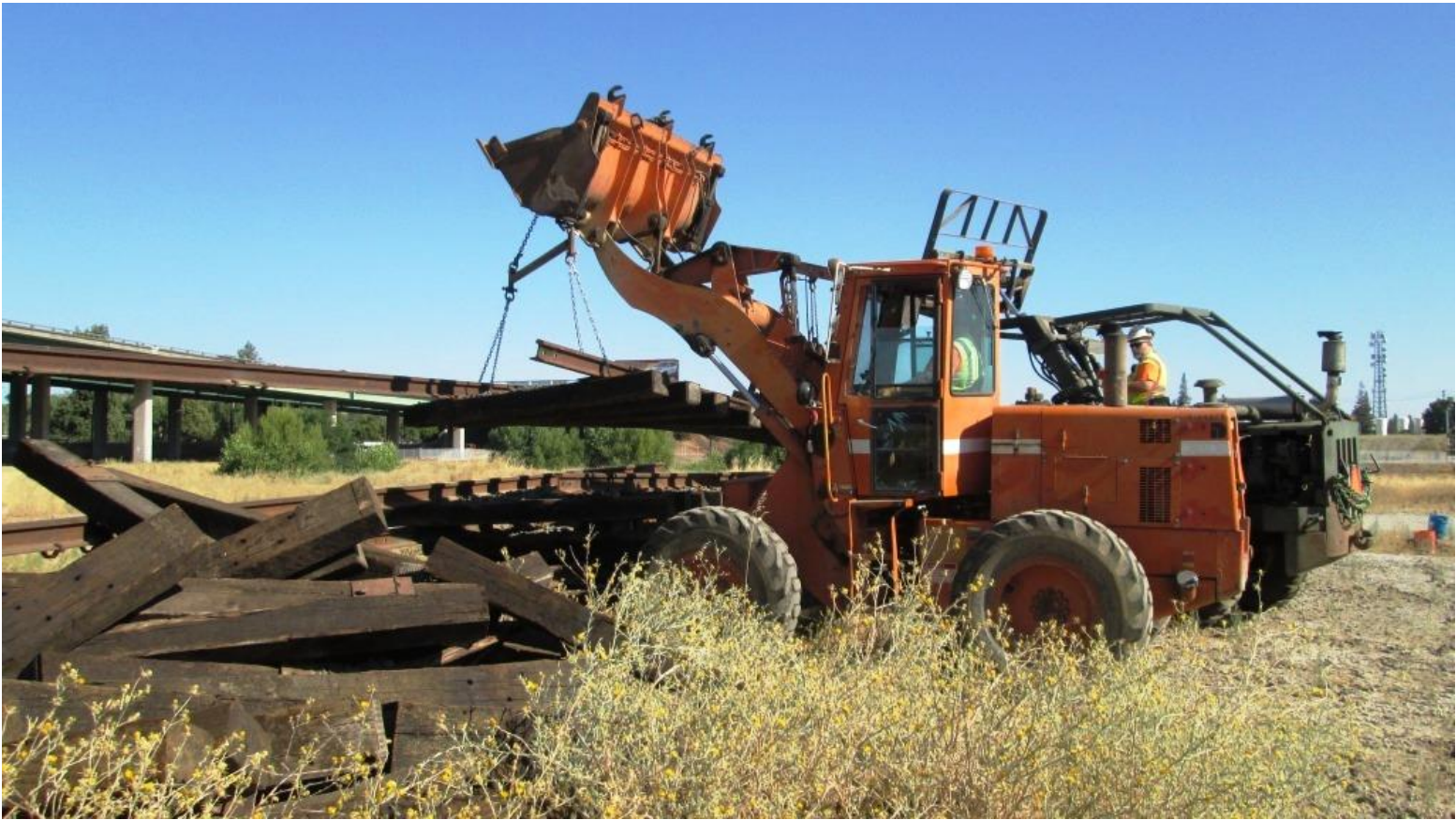
In a coordinated effort, Frank in the loader and Mike F. on Big Green move the first track-panel
