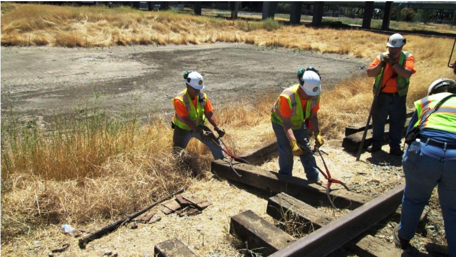
Joe and Mike W. pull that tie out
