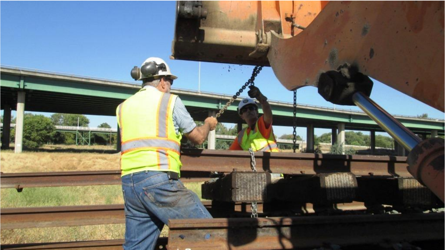
Alan and Joe chain the track-panel to the loader for lifting
