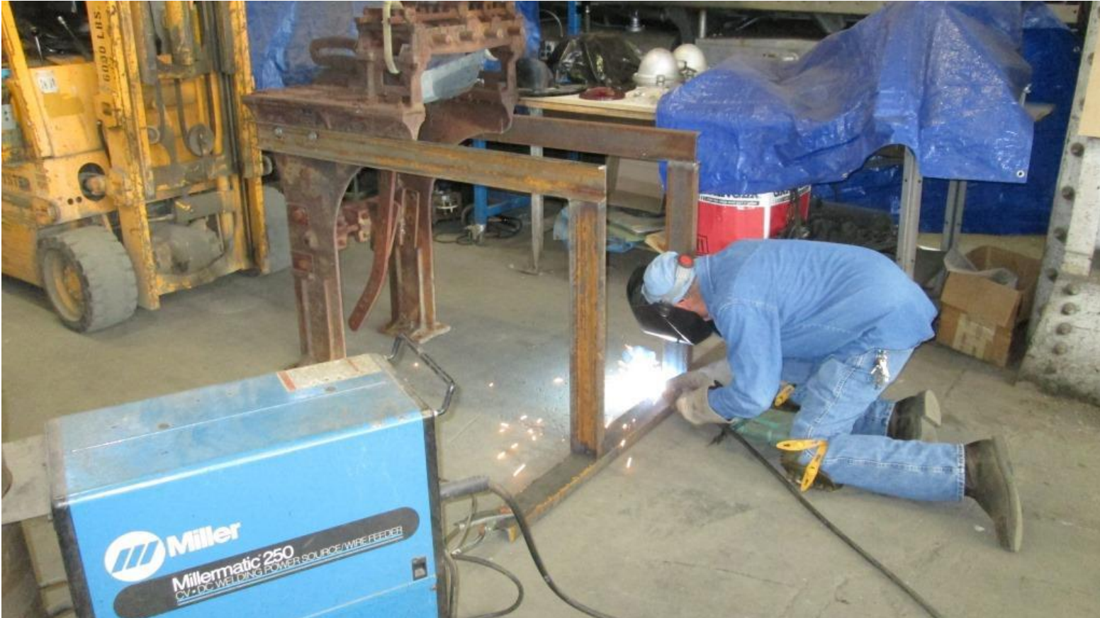
Cliff welds-up a stand for the interlocking mechanism being restored by the Signal Department
