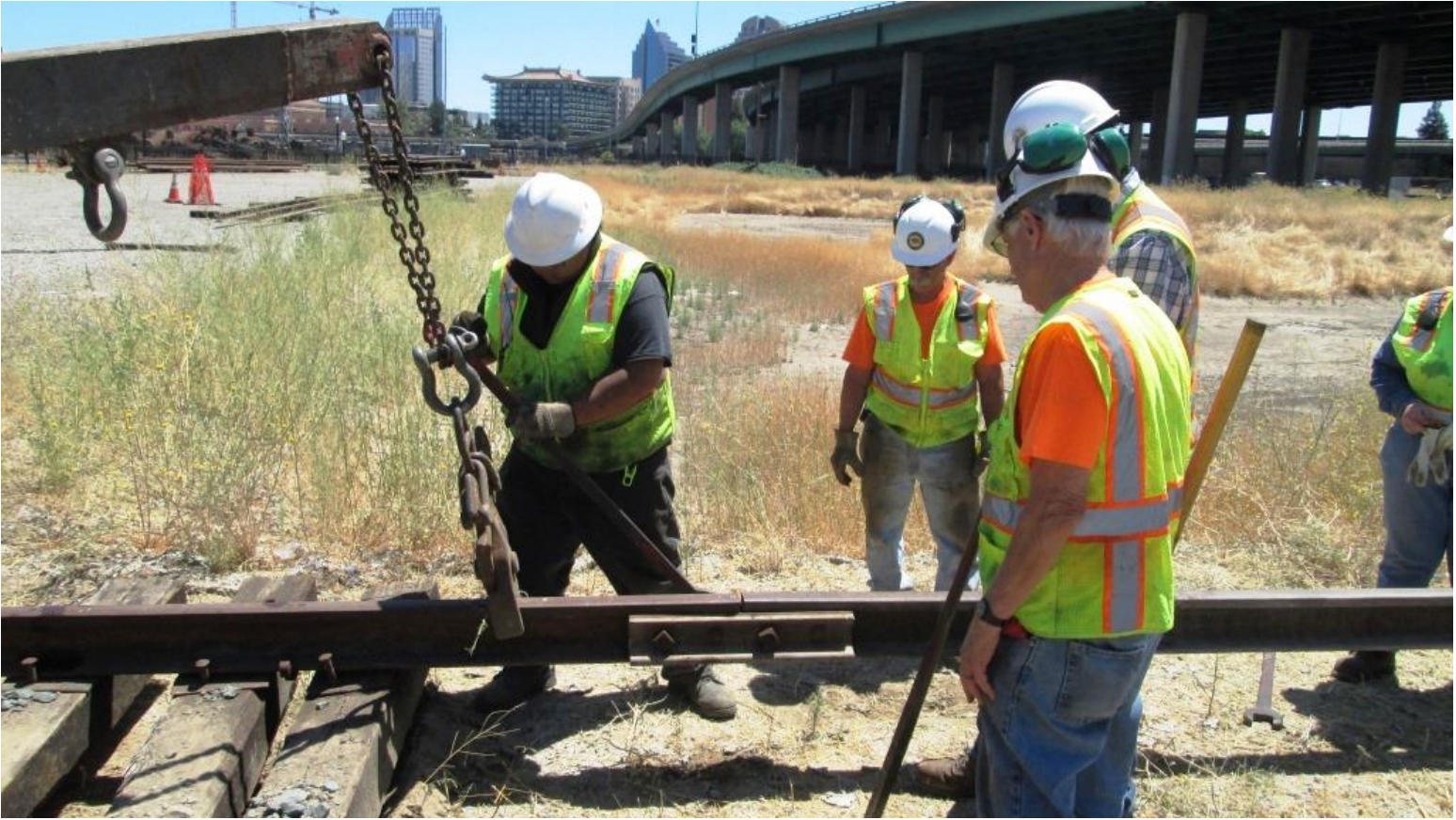
Anthony tightens down a bolt at the next joint
