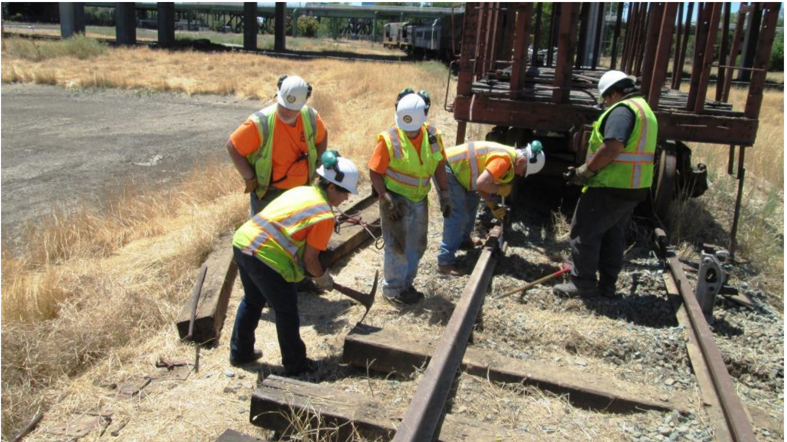
Pam digs around the next tie to come out as Mike W. and Anthony tighten down bolts
