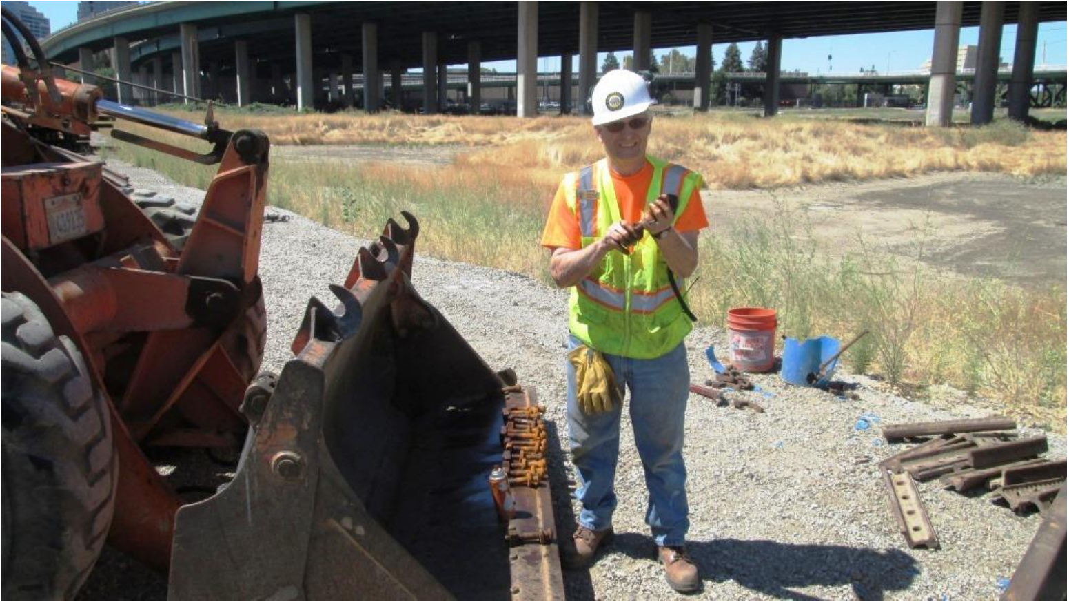
Mike W. oils and cleans rust off of the track-bolts
