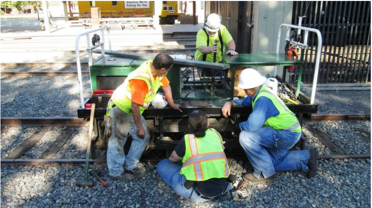
With the new rigging components in place, Frank tests the brake-stand
